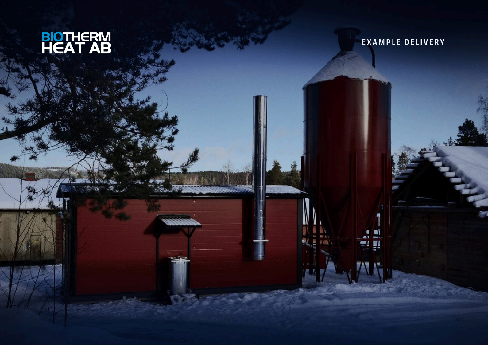
HEATING PLANT WITH PELLET SILO, CHIMNEY AND ASH CONTAINER
